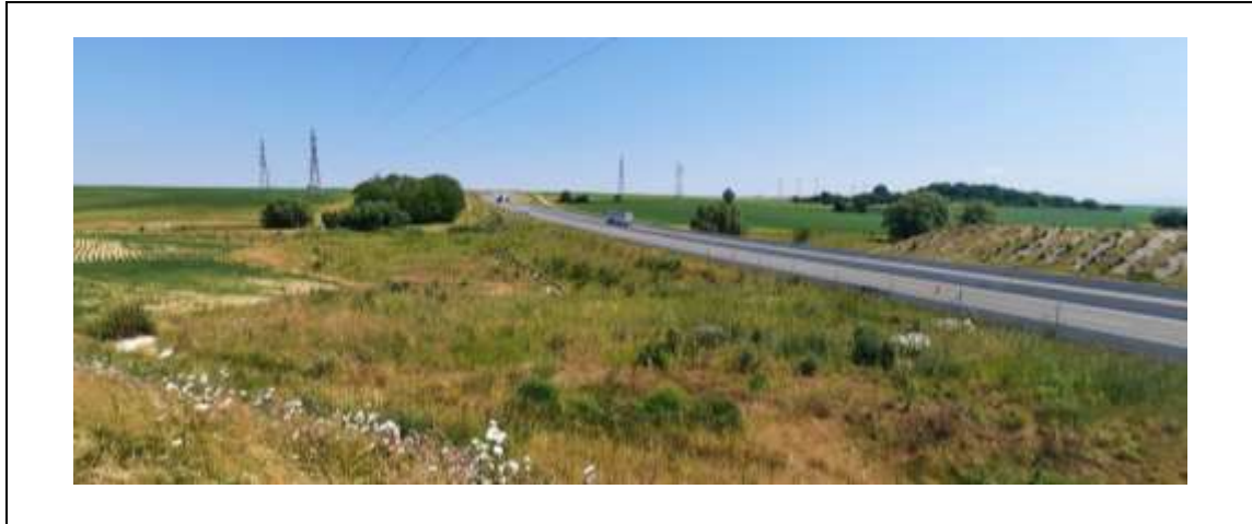
Figure 26. Sections of existing infrastructures can support experiments of hypotheses and solutions. Photo D. François, Université Gustave Eiffel.
