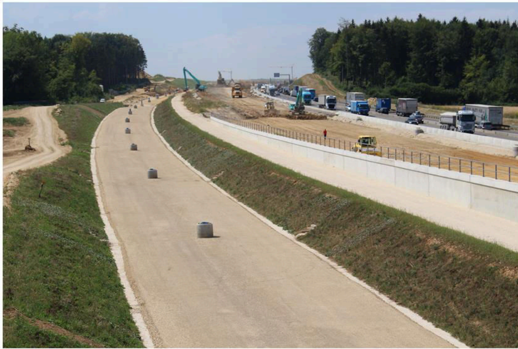
Figure 67: Bundling of a motorway with a high-speed railway Highlighting disproportionately high expenditure for bridges, maintenance and rescue routes, protective walls/concrete guards, separating strips, etc.
