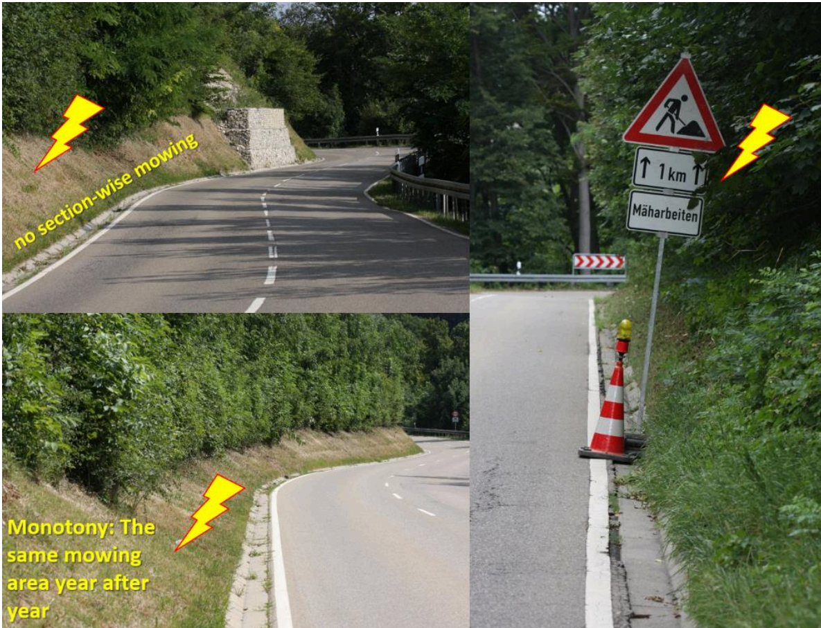
Figure 61: Serious maintenance errors on the Neuffen roadside
