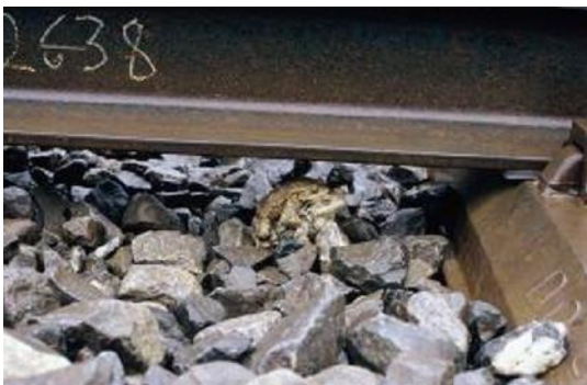
Figure 74: Deeply levelled ballast reduces Railkill of amphibians While tracks lying directly on the ballast or close to it are deadly barriers, deeply levelled ballast is a cost-free alternative that makes it possible for small vertebrates to cross railway lines. (Photos: E. Krummenacher in Rieder et al. 2006)
