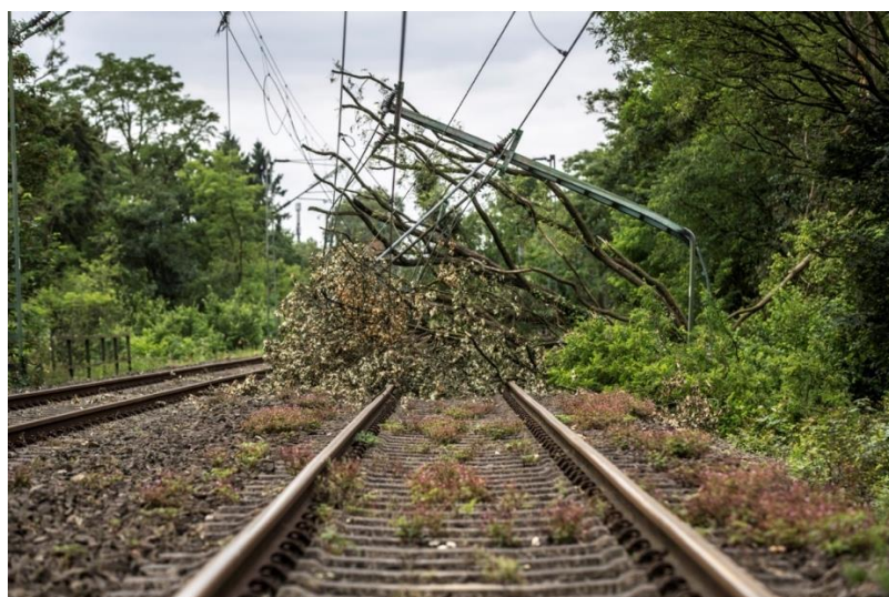
Figure 2-4: Rail tracks blocked by wind-blown trees and electric pipelines, Germany. Source: ©Michael Neuhaus/DB AG, provided by UIC.
