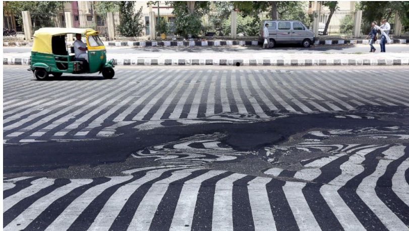
Figure 2-2: Melted road surface due to high temperature in New Delhi, India, on the 27th of May 2015. Source: ©Harish Tyagi/EPA
